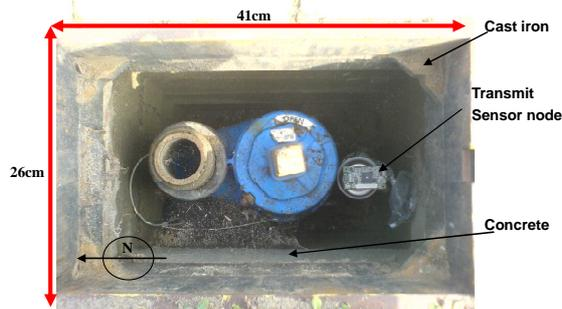
Fig.1 Structure of Fire Hydrant
